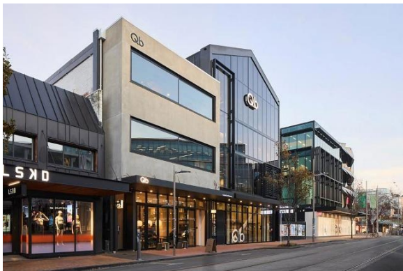
Qb studio building 235 – 237 High St
