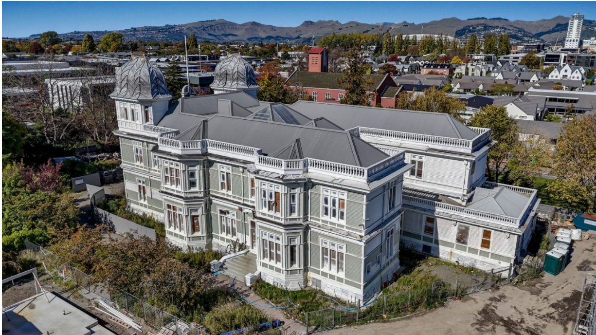
Aerial View of the exterior of McLean's Mansion
