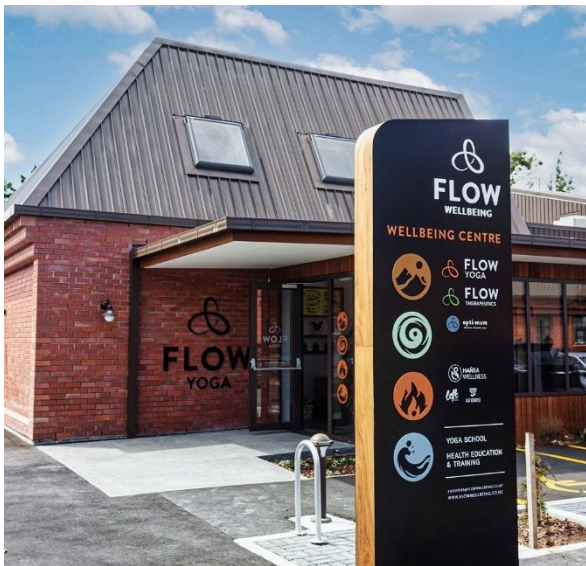
Entrance to 229 Fitzgerald Ave
