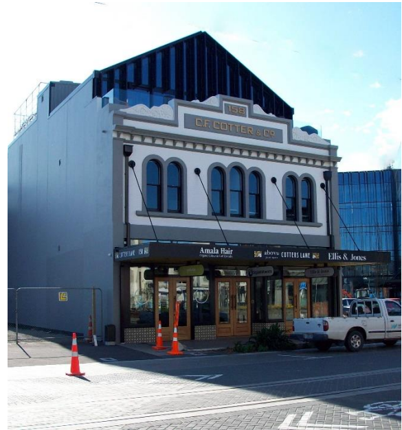
158 High St after restoration
