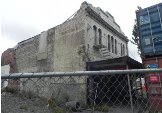
158 High St before restoration
