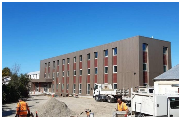
The new Te Koti Te Rato apartments, Rehua Marae
