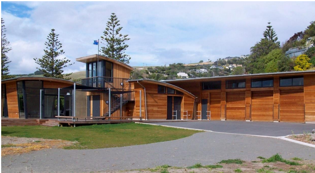
The new Sumner Surf Life Saving Pavilion
