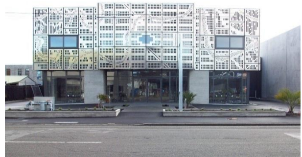
Corbel construction building, 213 Lichfield St
