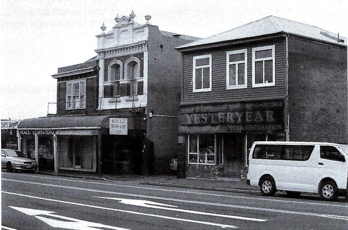
Heritage Shops 276 – 298 Colombo St Sydenham
