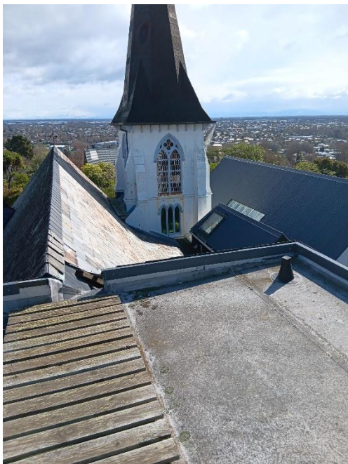
Ageing roof section of St Augustine's church
