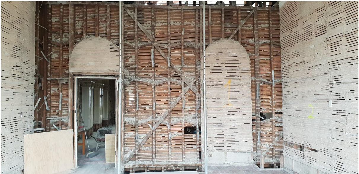
McLean's Mansion Upstairs where chimney brickwork has been completely removed
