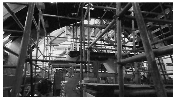
Interior work looking back to the chancel arch
